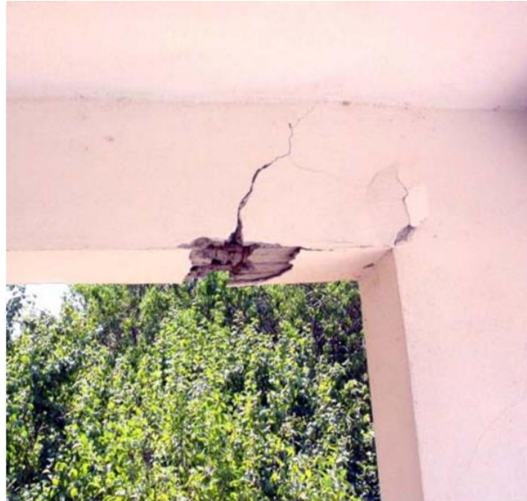
Damage severity 3
