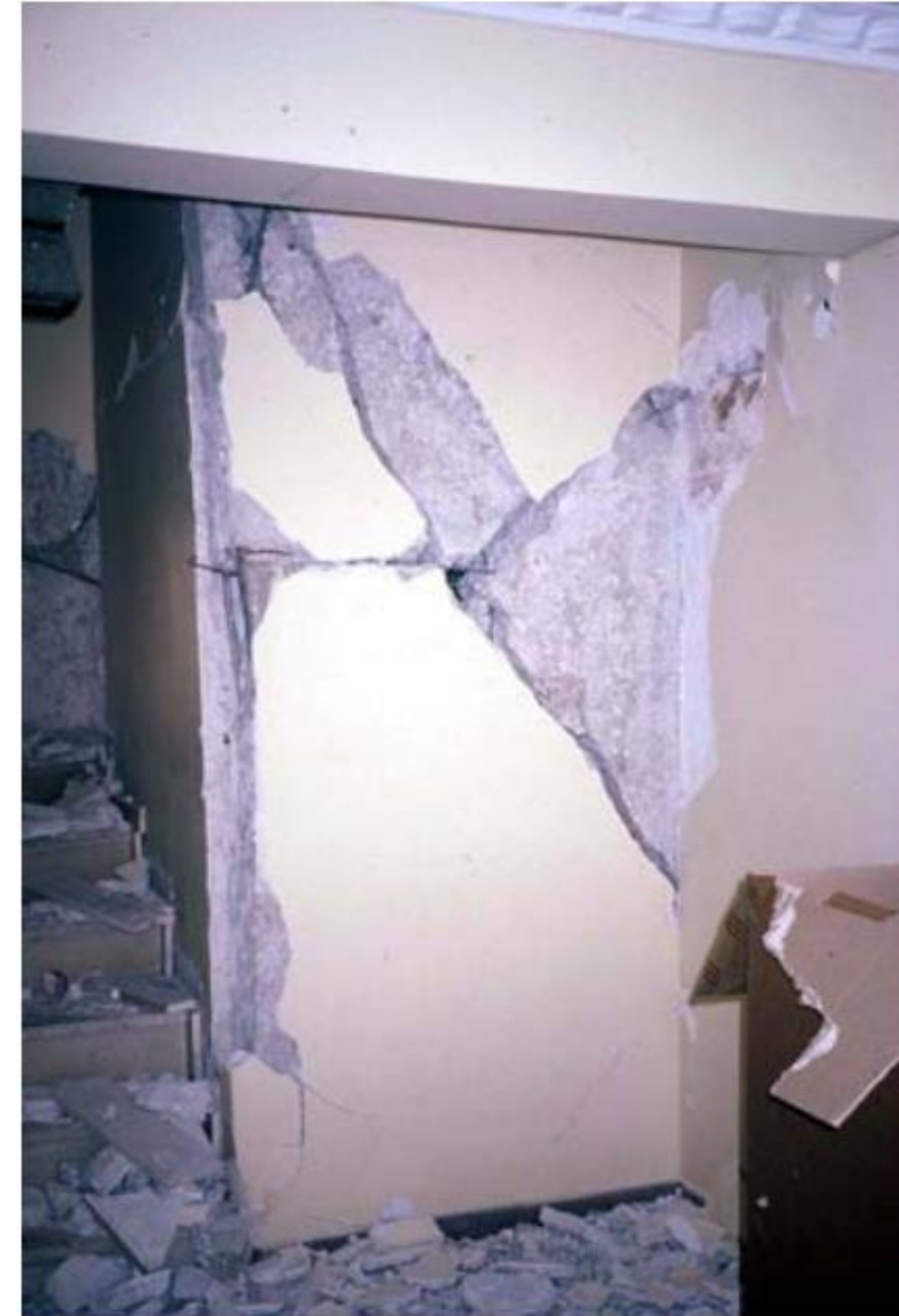
Damage severity 4
