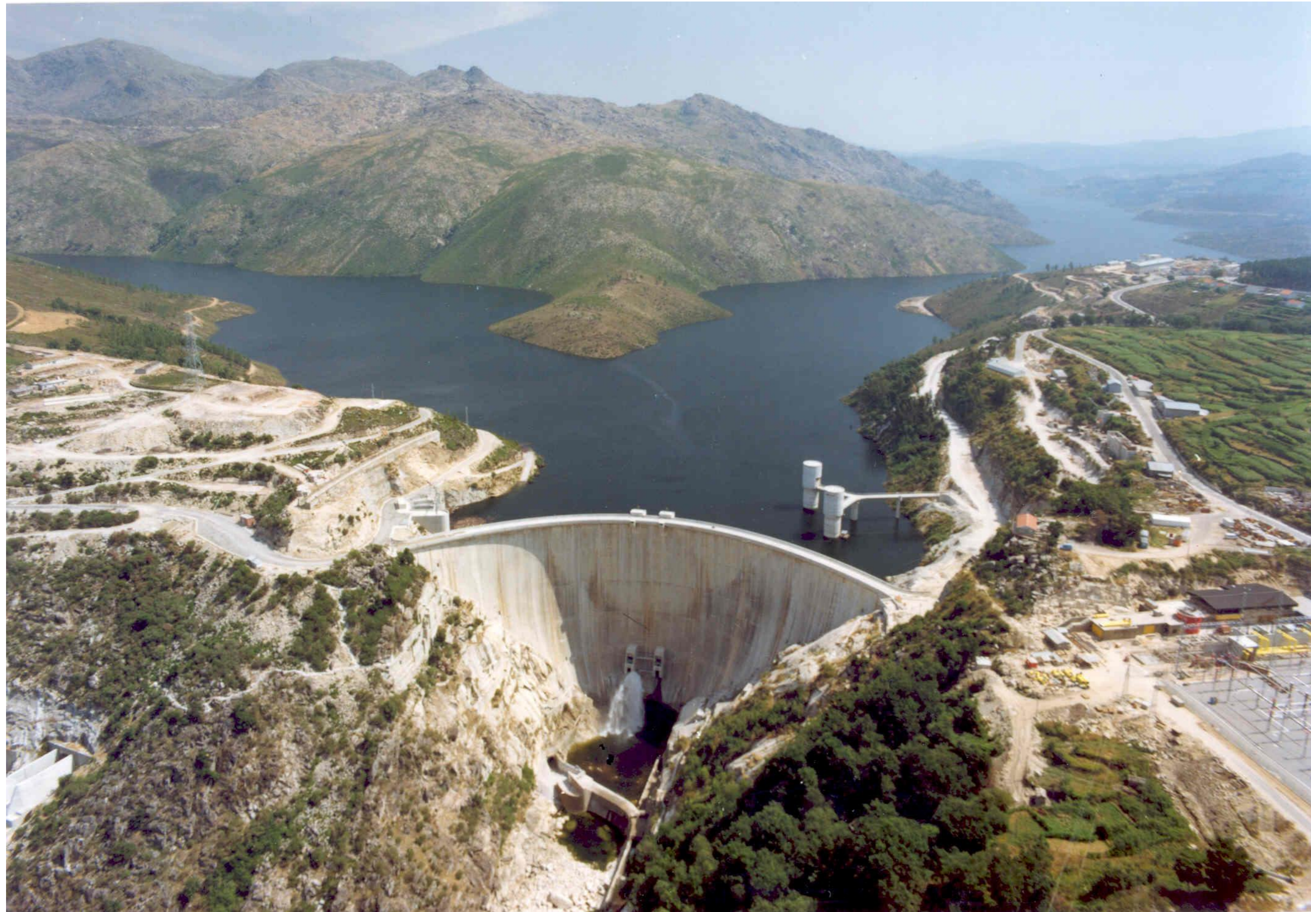
Alto Lindoso dam, Portugal
