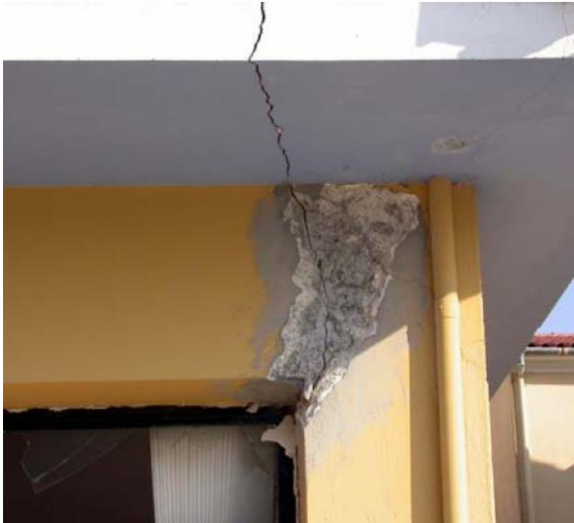
Damage severity 2
