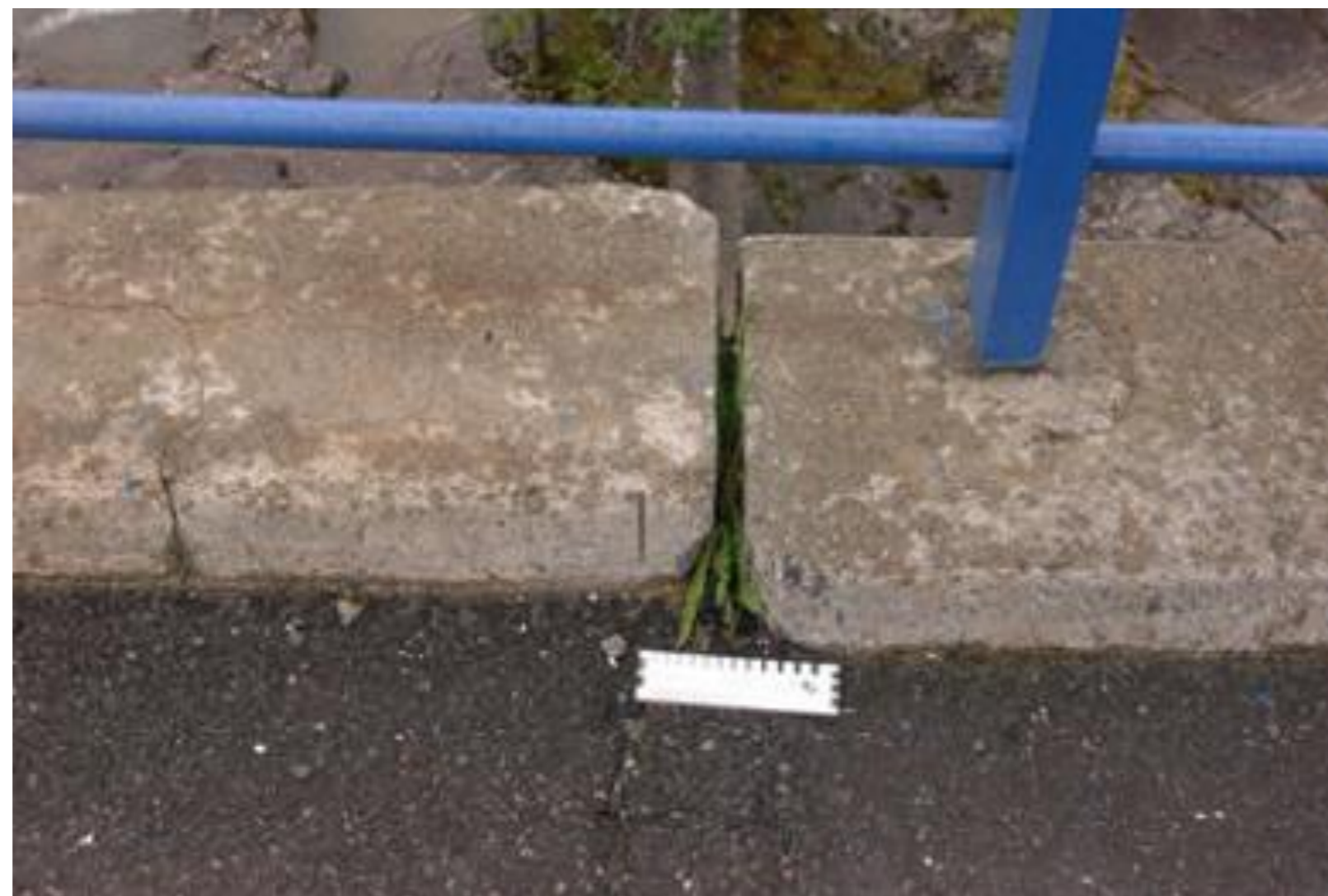
Misalignment in the crest of two different concrete dams
