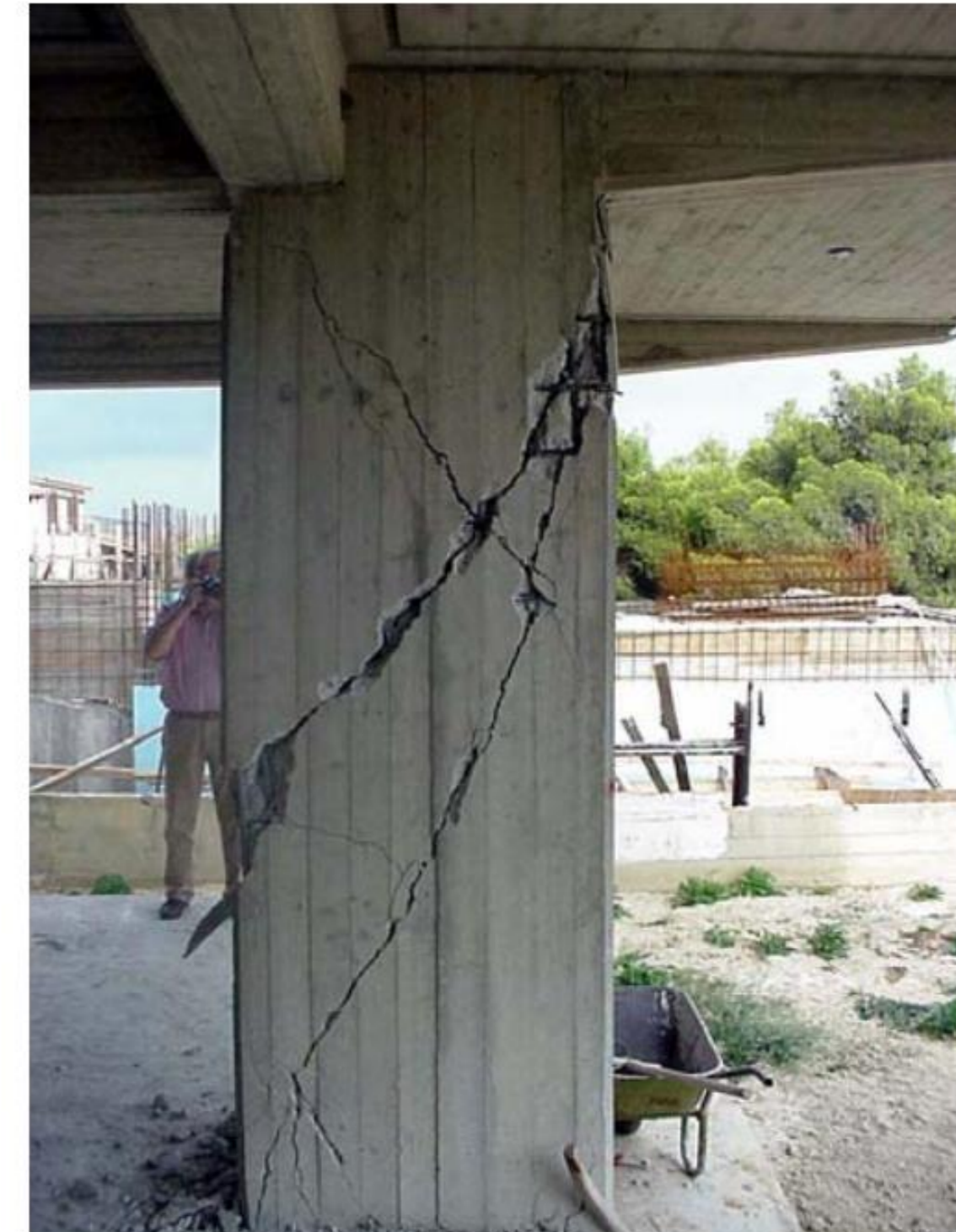
Damage severity 4
