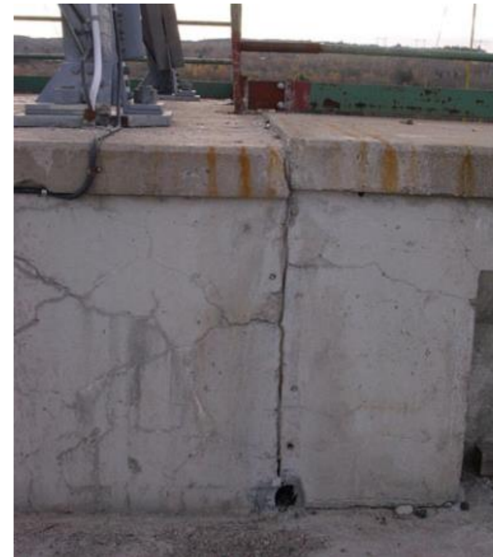
Misalignment in the crest of two different concrete dams
