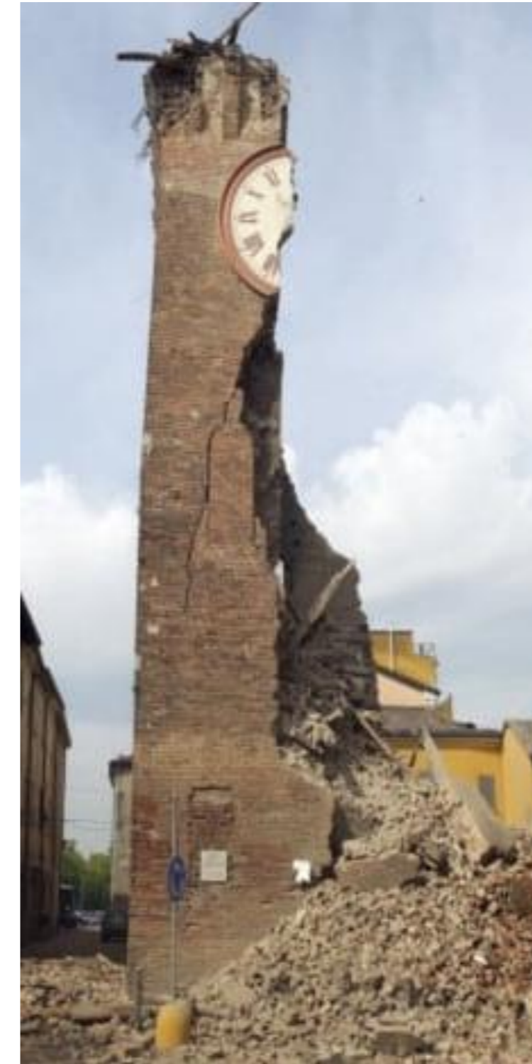
Vertical cracking
