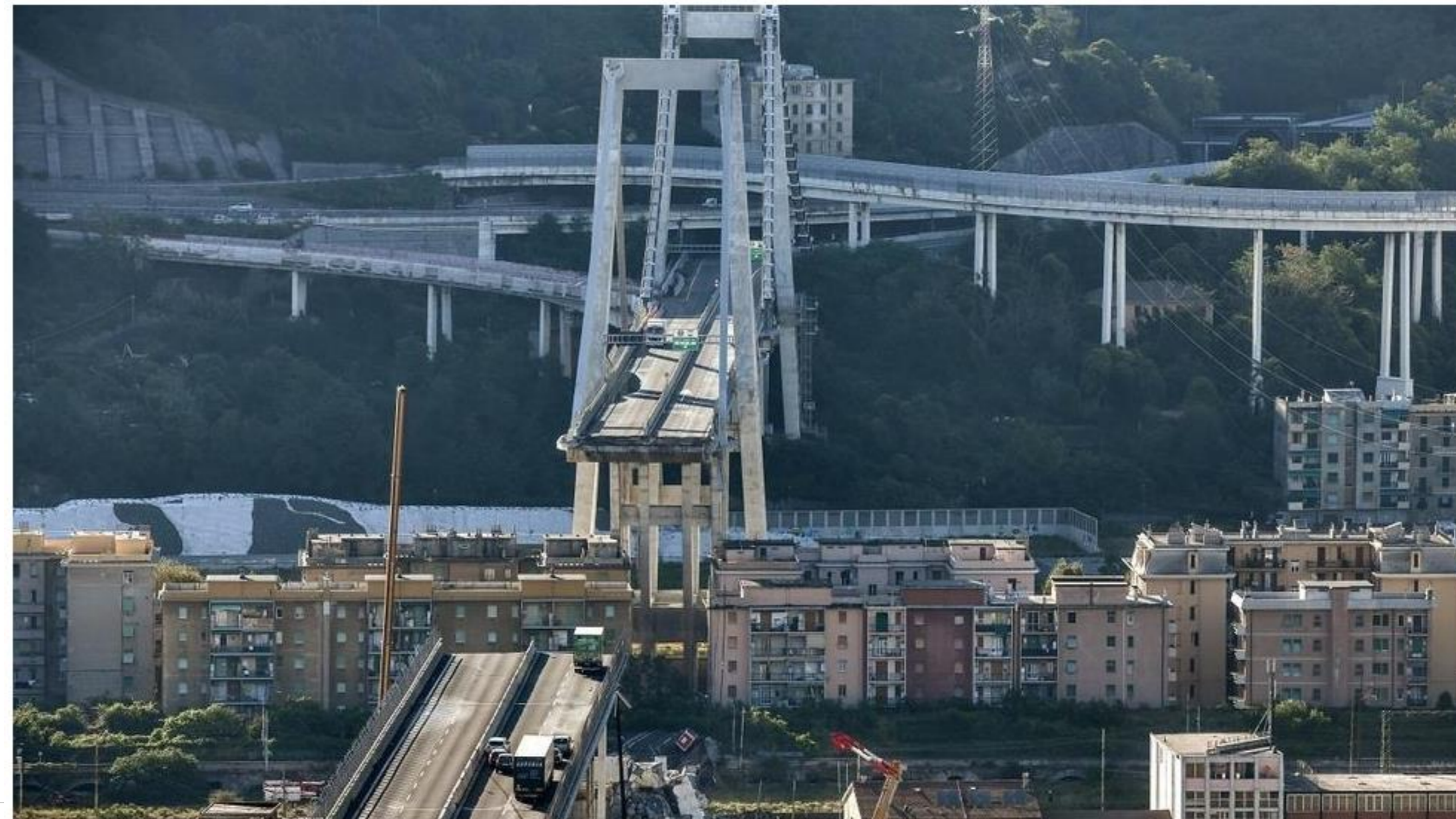
Piero Cruciatti, AFP | This general view taken on August 15, 2018, shows abandoned vehicles on the Morandi motorway bridge after a section collapsed in the northwestern Italian city of Genoa.
