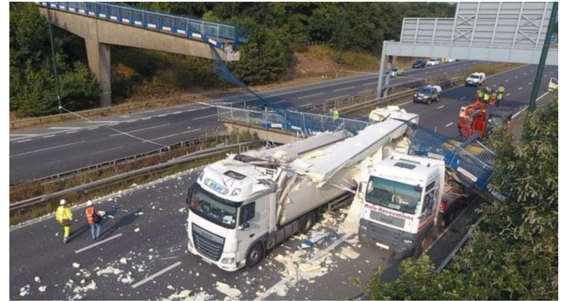
Lorry crash into a footbridge on the M20 motorway (Kent, 2016)
