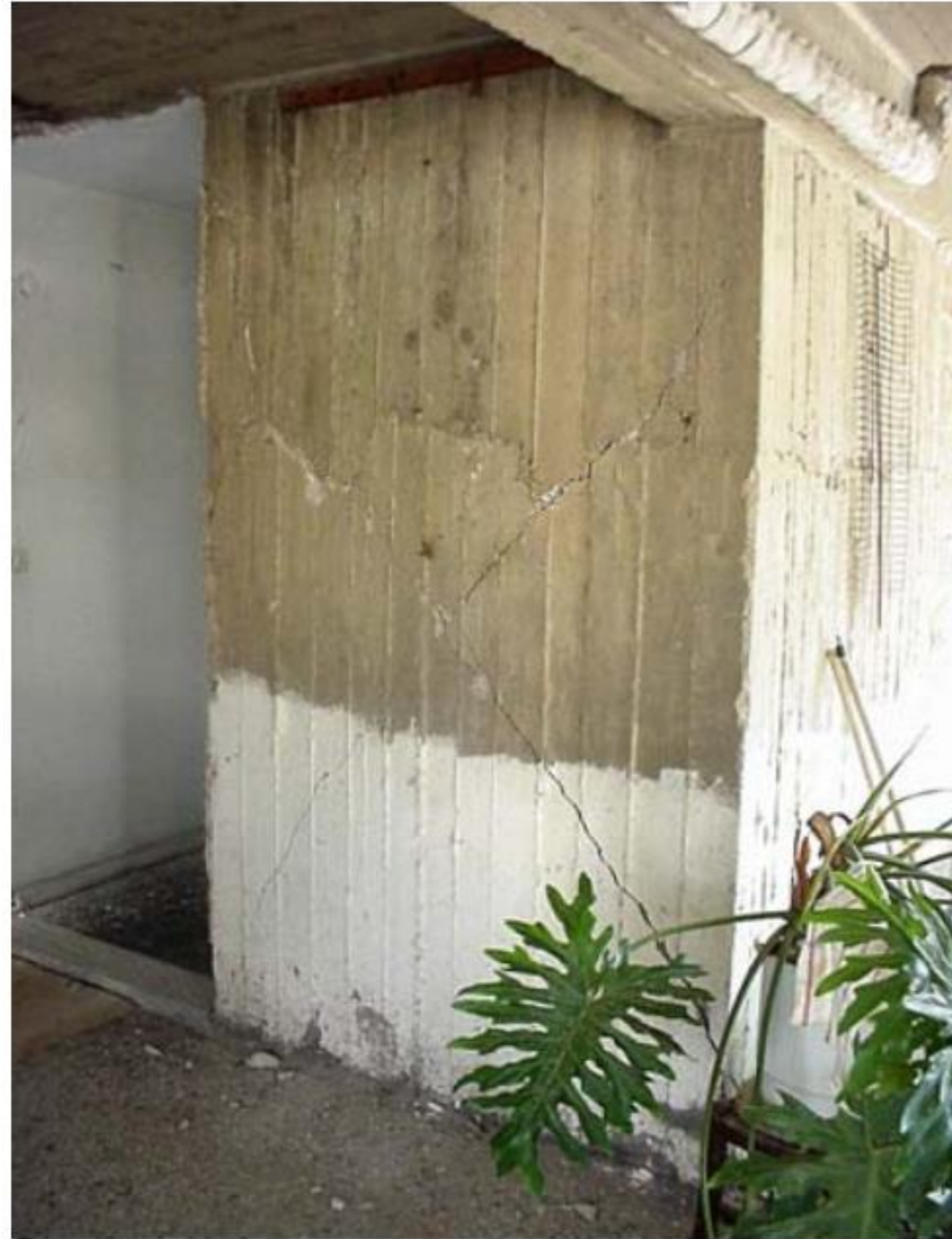
Damage severity 2-3
