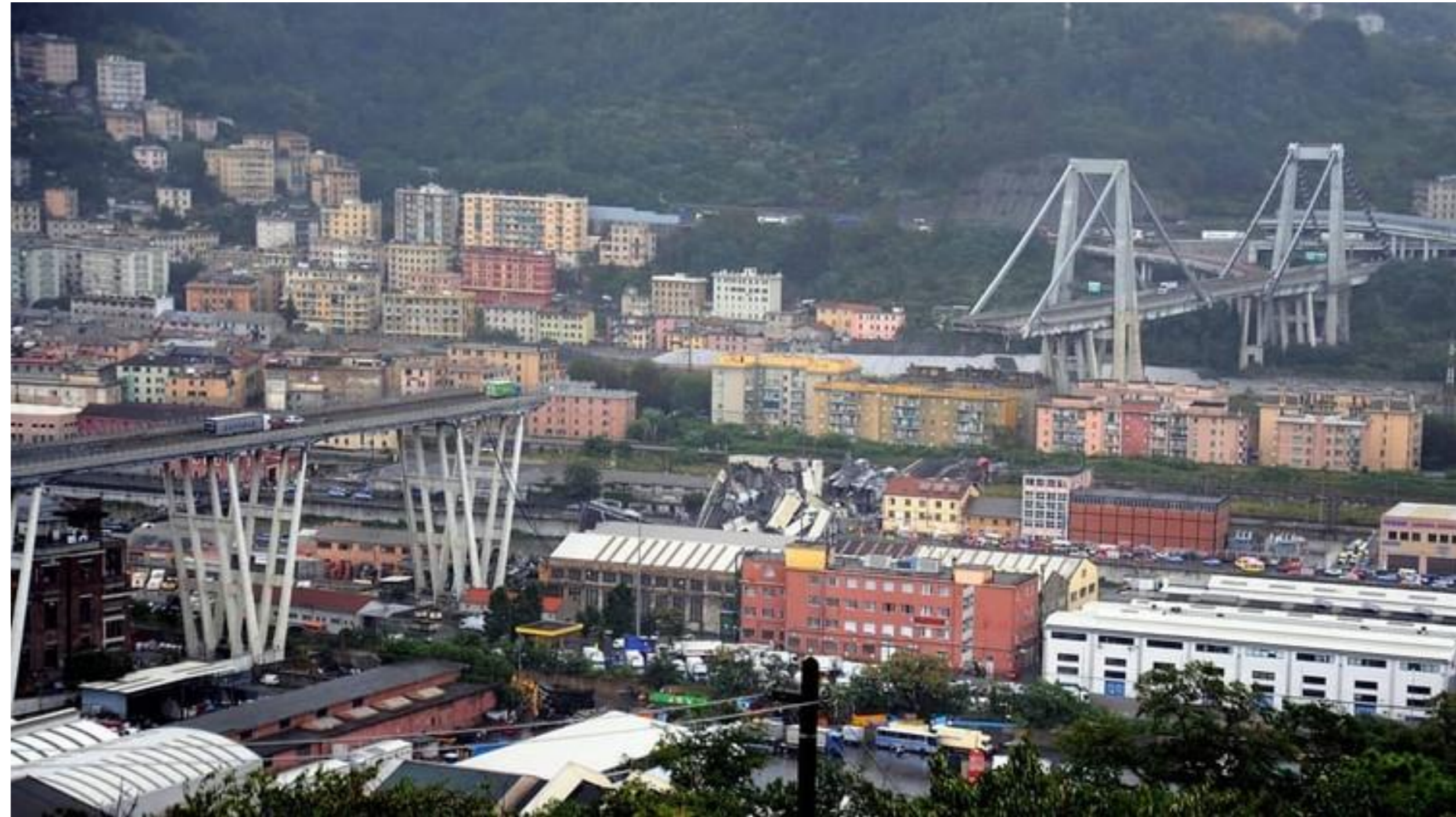
Morandi Bridge collapse (2018)
