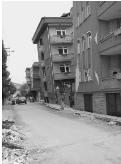
Figure 1.3: A 5-storey high building affected by liquefaction in Adapazari, Turkey (Bray et al., 2001)
