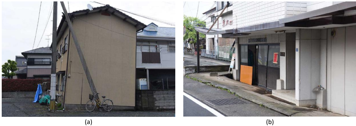
Figure 1.6: (a) Liquefaction-induced tilt of a 2-storey wooden house in Karikusa town; (b) Liquefaction-induced settlement of a 3-storey reinforced concrete building in Karikusa town (Tokimatsu et al., 2017)
