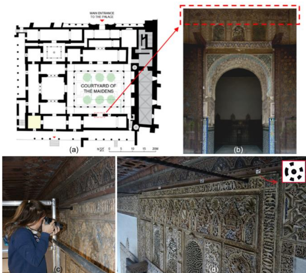
Figure 2: a) Ground floor of the Pedro I Palace (RAS); b) General image of the main entrance to the room of the ceiling of Charles V; c) On-site work; d) Details of the frieze under study and targets used.
