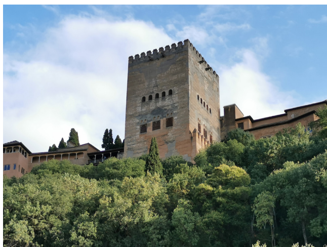
Figure 1. External view of the Tower of Comares.
