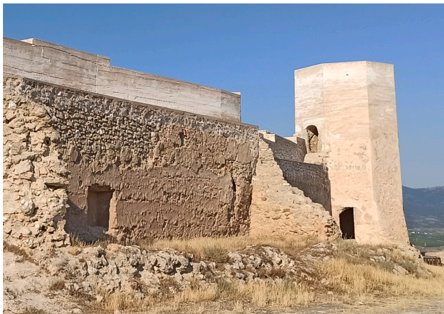
Fig. 1. Ayyup Castle (Aragon, Spain) built in the 9th century using gypsum blocks and mortar.
