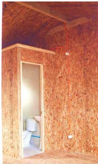
Figure 6. Sanitary module of Prototype House by TecnoPanel, Onemi and CIGIDEN. Source: [41].
