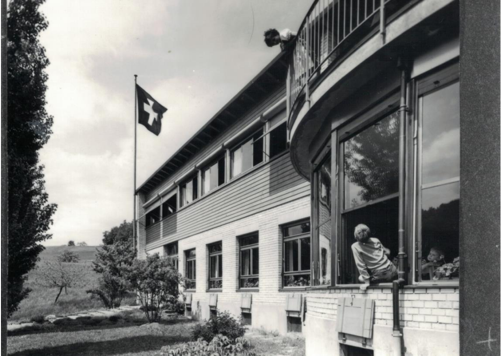
Figure 7: Hannes Meyer, Kinderheim in Mümliswil, view of the southern facade (Archiv gta-ETH, Zurich).
