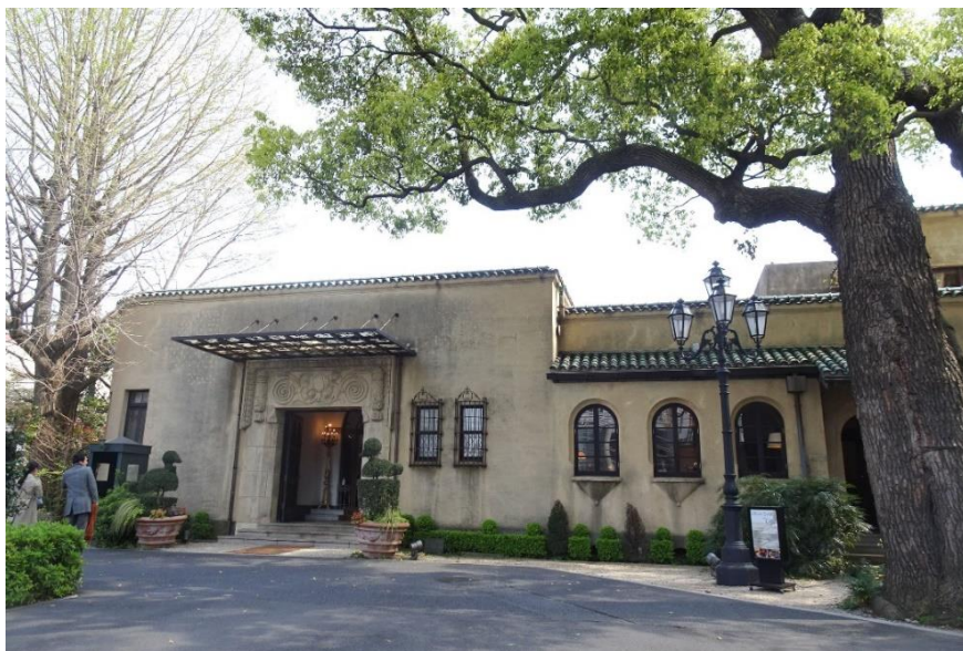
Figure 2: Seiichiro Chujo and Tatsuzo Sone, Count Ogasawara Residence in Tokyo, 1927 (Author's photo in 2020).
