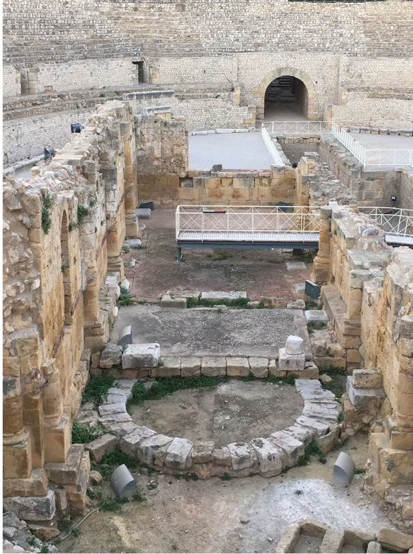
Fig. 2 Christian basilica built on top of the Roman amphitheatre in Tarragona. The standing structure is high medieval, but excavations have shown the foundations of an apsed basilica underneath, dated to the sixth century. Photograph by the authors [Colour figure can be viewed at wileyonlinelibrary.com ]
