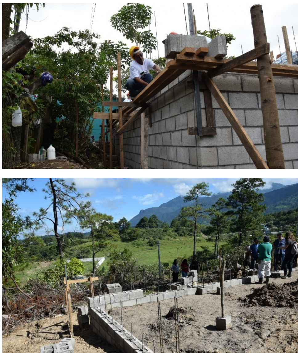
Figure 7. Construction of the prototypes in Jocoaitique and La Palma.
