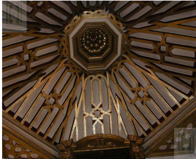
Fig. 89. Charpente octogonale dite du Chapetón (1 er quart du XVII e siècle). Juan Guillermo Moncada, 2012 http://spoliarium-macellum.blogspot.com/2012/06/iglesia-san-francisco-de-bogota.html
