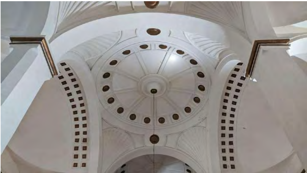
Figure 209: Top: Interior ceiling in the church of Mancha Real. Bottom: Spherical vaults cover the central nave. Detail of a spherical vault covering the central nave of Valdepeñas de Jaén. © Manuel Sánchez García, 2020.
