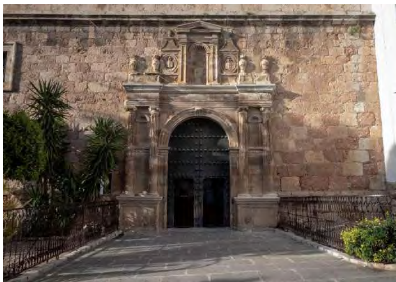
Figure 207: 1572, Lateral façade of Mancha Real's main church, projected by Andrés de Vandelvira. The white wall on the right belongs to the priest's house. © Manuel Sánchez García.
