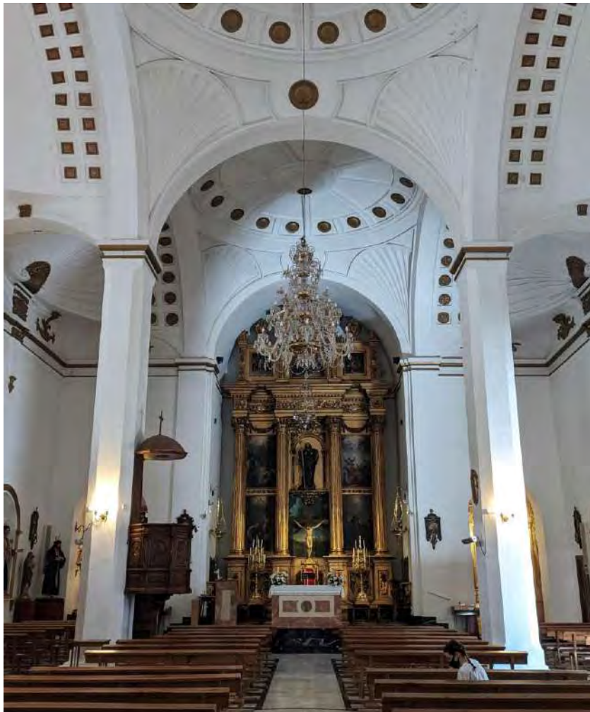
Figure 208: Top: Interior of the church of Mancha Real. Bottom: Interior of the church of Valdepeñas de Jaén. Both buildings share several architectural characteristics. The main common element is the spheric vault, typical in the architecture of Andrés de Vandelvira and other renaissance works in Jaen. © Manuel Sánchez García, 2020.
