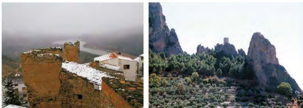
Figure 108: Torres de Orcera (top), Castillo de Hornos (bottom left) and Tower of Castellón de Figue (bottom right). Photos by Silvia Fernández Cacho, 2010. © Junta de Andalucía. 436
