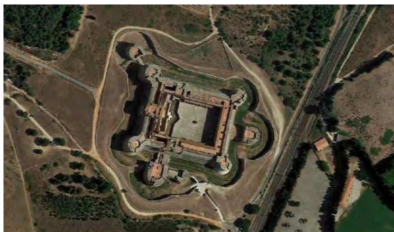
Figure 100: Satellite view of Salses Fortress, Roussillon, France. Its layout was modified by Ramiro López in 1496 by order of king Ferdinand II of Aragon. The east and south bastions were added at that point to the pre-existent fortress. © Google Earth
