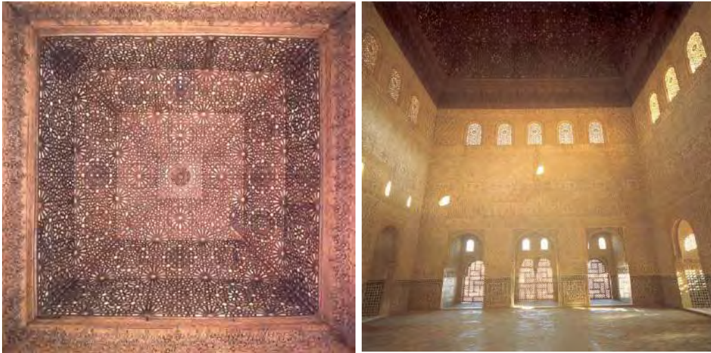
Figure 93: Ambassadors Hall in the Alhambra. Left: Wooden lace ceiling. The octagonal stars of each layer aligned in the vertexes, forming four tree-like structures that meet in the central star. Right: General view. The throne was placed in the central double niche, oriented to the north and overseeing the city of Granada. ©Architectural Composition Department, Universidad de Granada.
