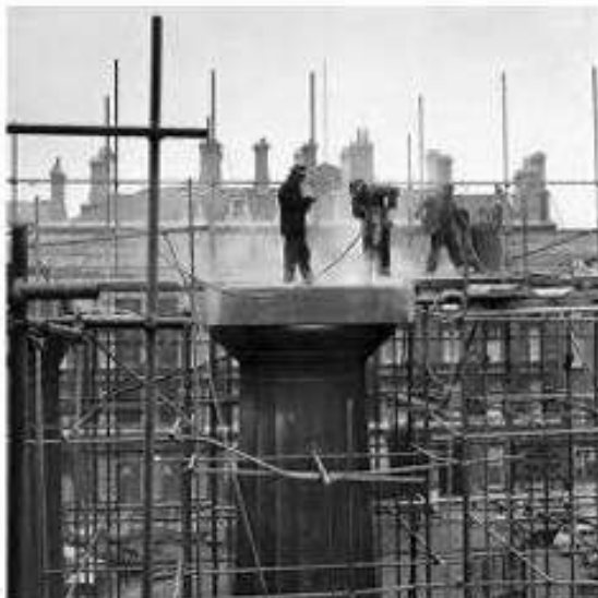
Figura 4. Demolition of the 124 year old, doric-style arch at Euston Station, London, 1962
