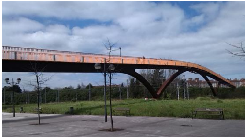
Figure 1. The Pumarín-Moreda footbridge
