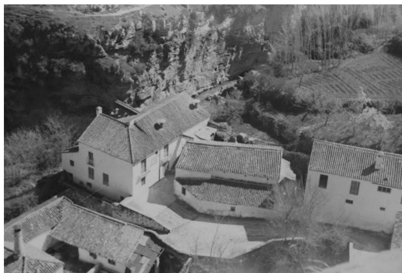
Figure 28. Fábrica de Harinas la Purísima in 1963, next to the Tajo y Alhama River [17].
