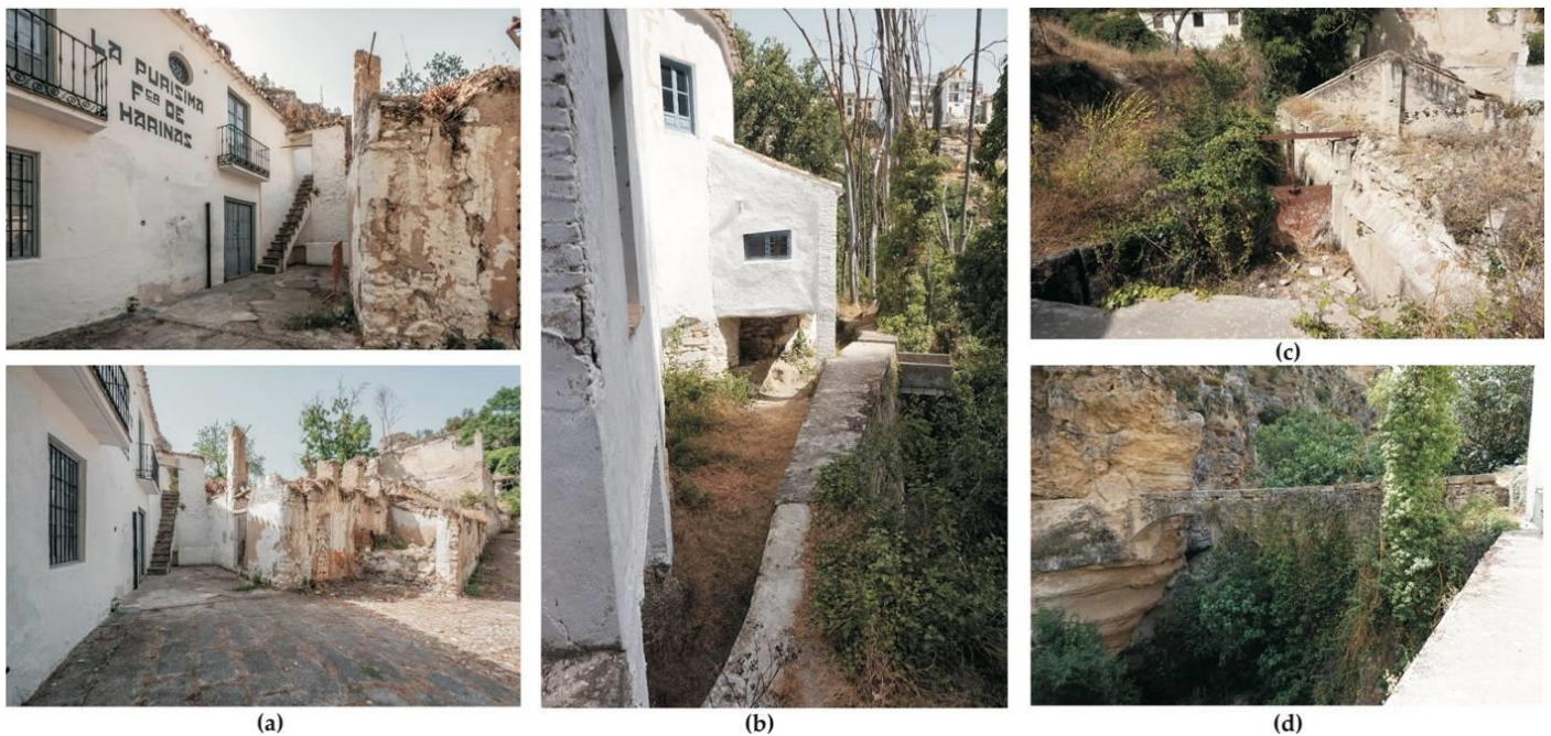
Figure 22. Photographic documentation of the exterior of the Fábrica de Harinas la Purísima: (a) facade of the main building and the stable in ruins (J.G.M.-S.); (b) rear facade with the Caz del Molino ditch and overflow towards the Marchán River (M.d.C.V.-L.); (c) metal gate in the Caz del Molino ditch next to the stable (M.d.C.V.-L.); (d) 16th century aqueduct next to the mill (M.d.C.V.-L.).
