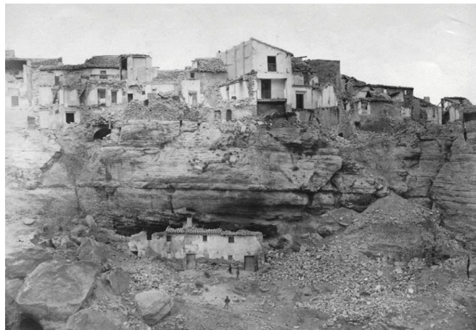
Figure 15. Photograph taken after the 1884 earthquake of a sunken house on the edge of the Tajos [54].
