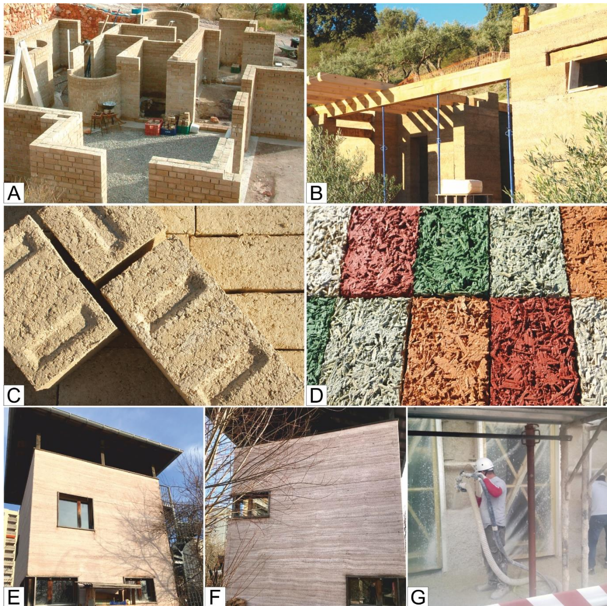
Fig. 1. Hemp concrete constructions built with premade building blocks (A) and cast, compacted loadbearing, hemp-clay concrete walls (B). Building blocks made from hemp shives (2-25 mm) and a clay binder (C) or hemp shives (2-25 mm) and a lime binder, with or without addition of mineral pigments (D). (E) and (F) show different views of a building made with non-loadbearing, casted hemp-lime concrete walls after 20 years exposure to weathering conditions in Switzerland. (G) Sprayed application of hemp concrete as an outer coating.
