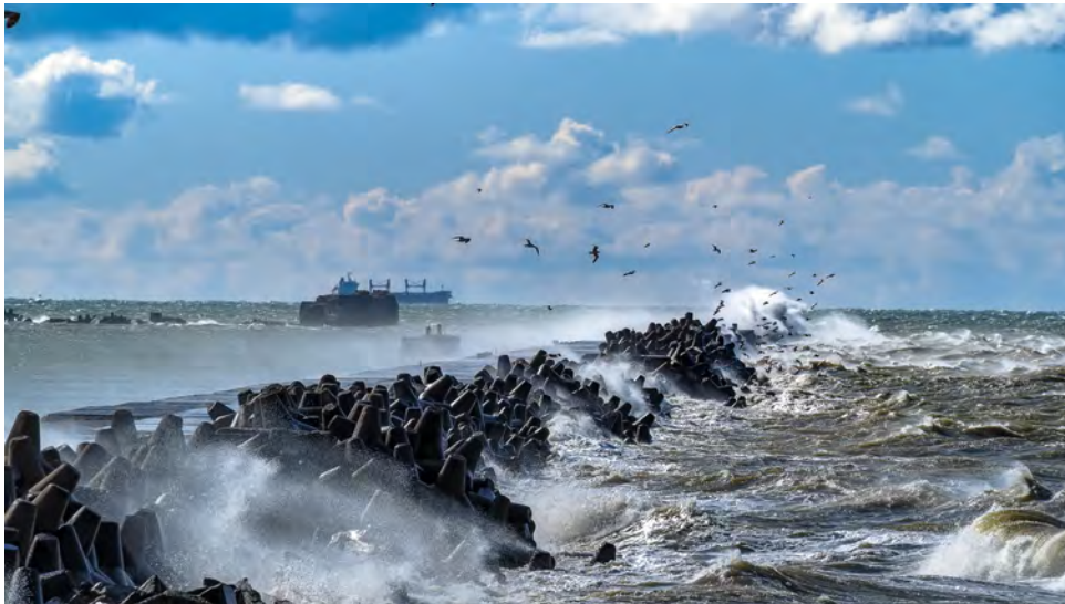
FIGURE 1.1: Different run-up heights on a rubble mound breakwater with crown wall and overtopping due to a higher run-up.
