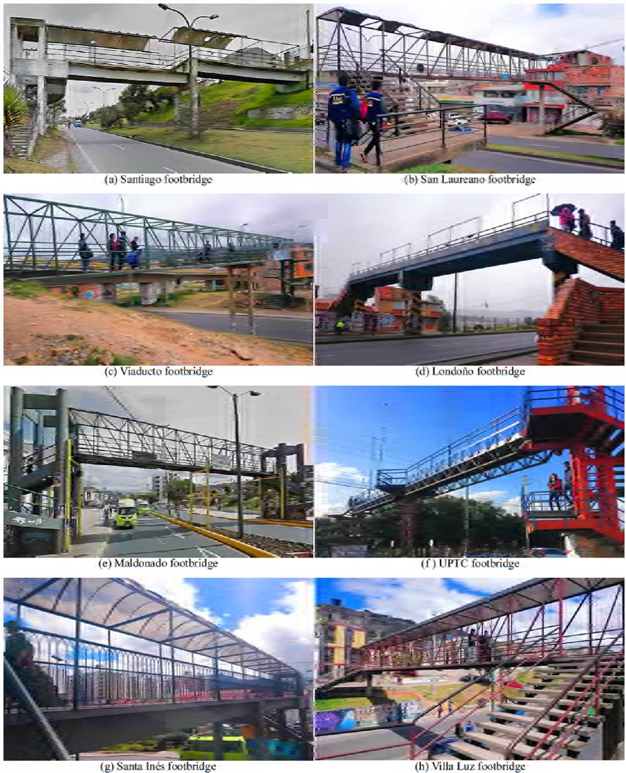
Fig. 2. General view of the studied footbridges
