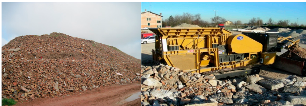
Figure 5. Examples of construction and demolition waste (CDW) management. On the left, unsorted cumulus of materials from emergency management in the event of the Emilia earthquake (2012; on the right, a mobile CDW treatment plant.
