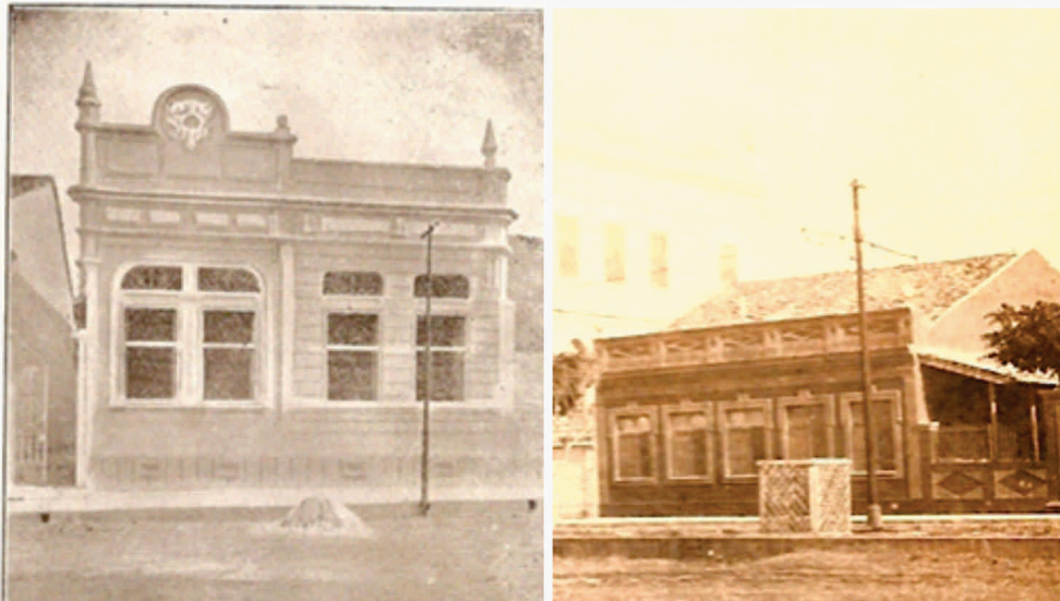
Figure 5: Photographs of residential dwellings with boundary walls Source: Digital collection from the Public Archives of Alagoas (APA)
