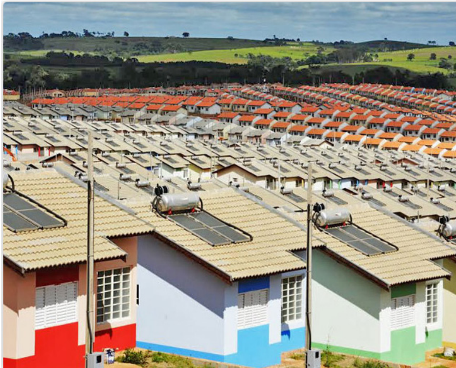
Figure 4: Photograph of João Domingos Netto Housing Complex, Presidente Prudente Source: Particular collection
