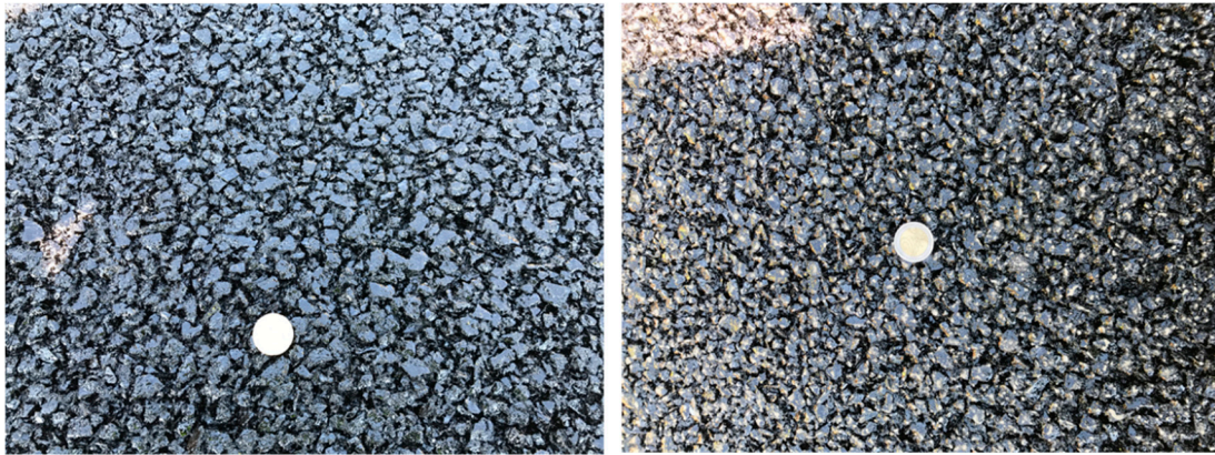
Figure 15. Visual appearance of the CRMB-HMA (left) and CRMB-WMA (right) after compaction.
