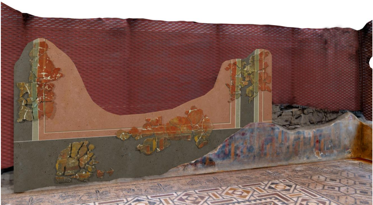
Figure 5. Final image rendered image of the room, including the chromatic reintegration of the intervention mortar.
