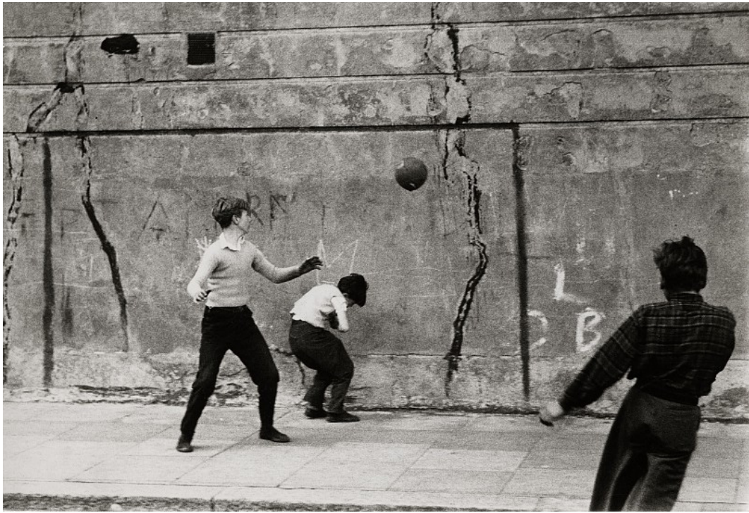
Fig. 14 - Roger Mayne. Southan Street, North Kensington . Londres, 1956. En gittermangallery.com
