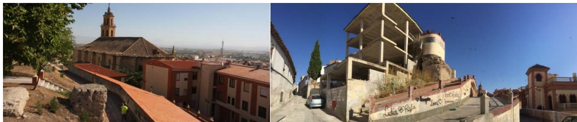
Figures 2-4. (2) West Border: Rear of houses and view of part of the Cloister of S. Francisco, (3) Cover of the row of garages and in the background the tower and roofs of the Main Church, (4) Unfinished work: Structure of reinforced concrete on remains of the wall of the Alcazaba. Source: Photos of F.J. Lafuente and own elaboration
