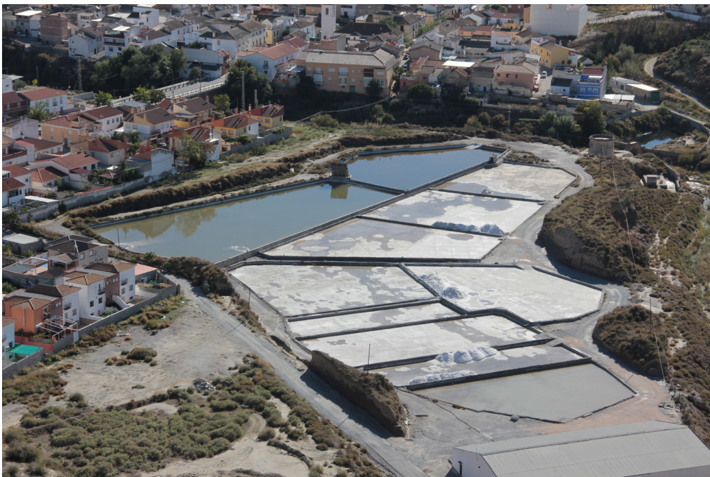
Figure 30. The “salina” (solar salt pond) of La Malahá. The Roman Tower, seen at the upper right-hand of the picture, is very close to the point where the saline-water spring locates. The saline water, which pours into the “Río Salado” river, is then pumped into the “salina”, placed a couple of metres higher than the river bed.
