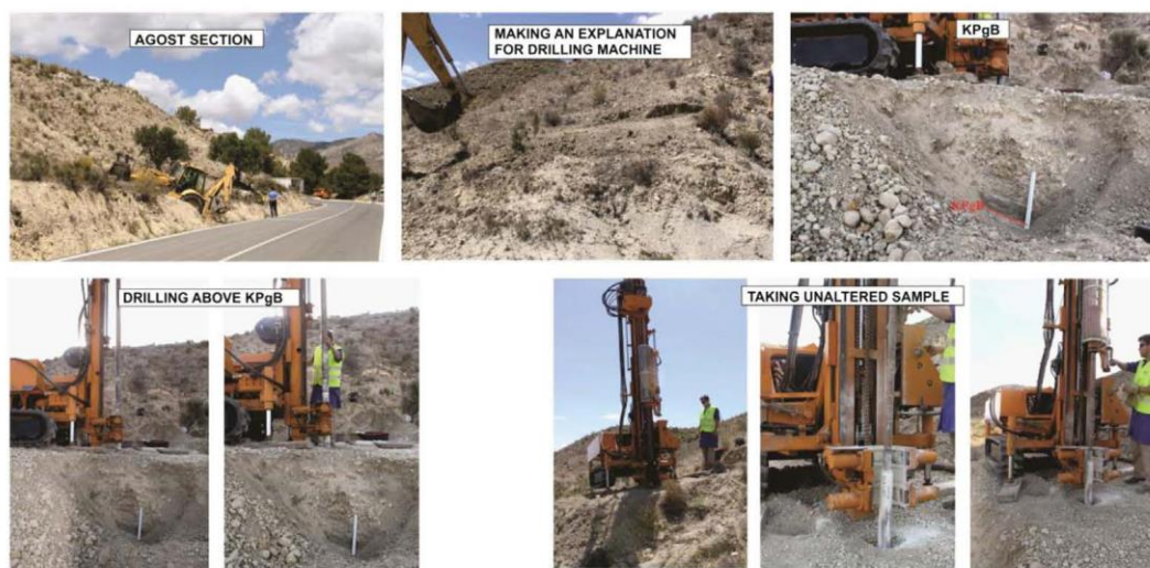
Fig. 1. Photographs of the Agost site, during the drilling and unaltered sampling.
