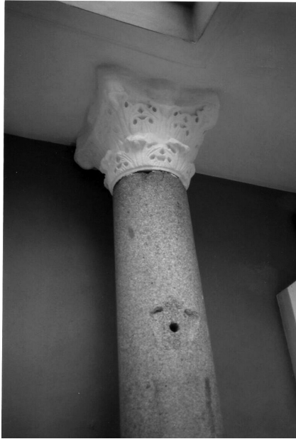
Fig. 11: Kırkçübaşı mosque, column and capital of the portico
