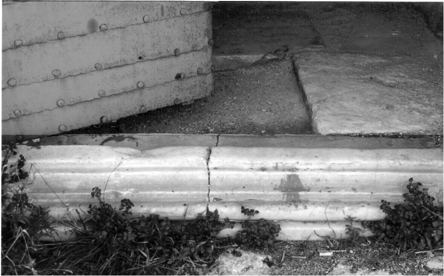
Fig. 1: Yedikule, threshold of a door
