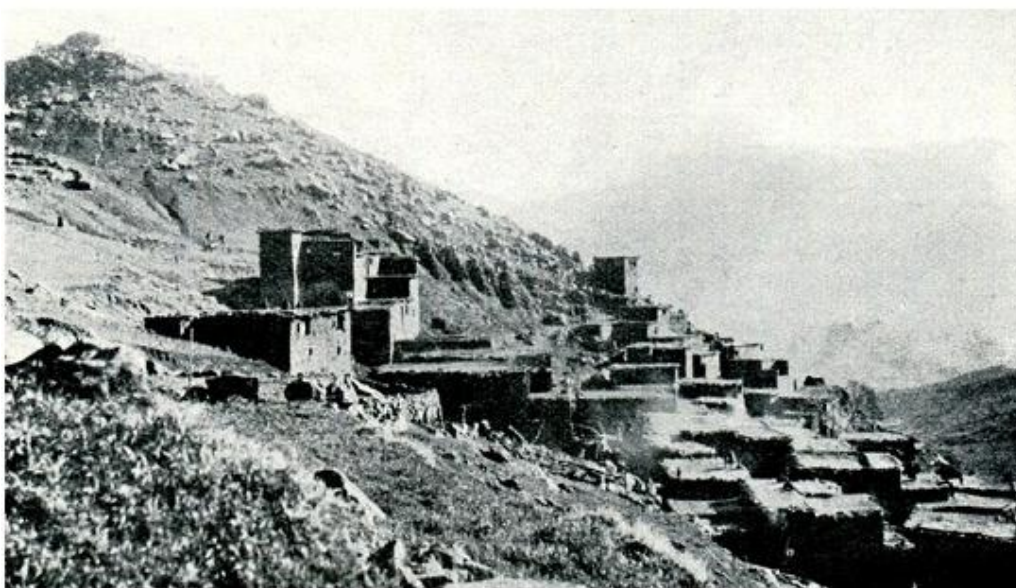
Figure 11: Rural architecture in precolonial Morocco
