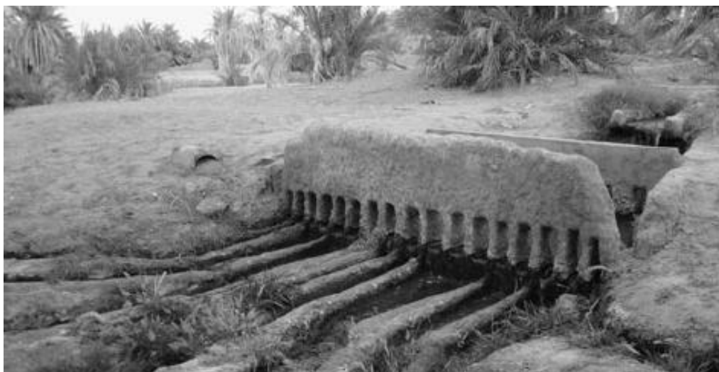
Figure 8: Flow splitter to distribute water shares
