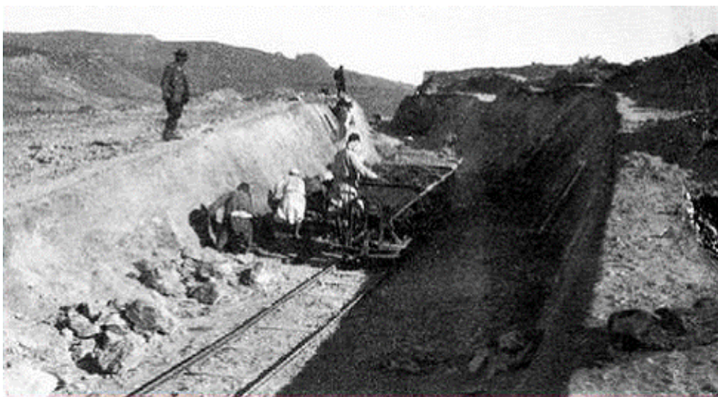
Figure 34: Construction of the Melilla-Uixen railroad for the purpose of mineral exploitation
