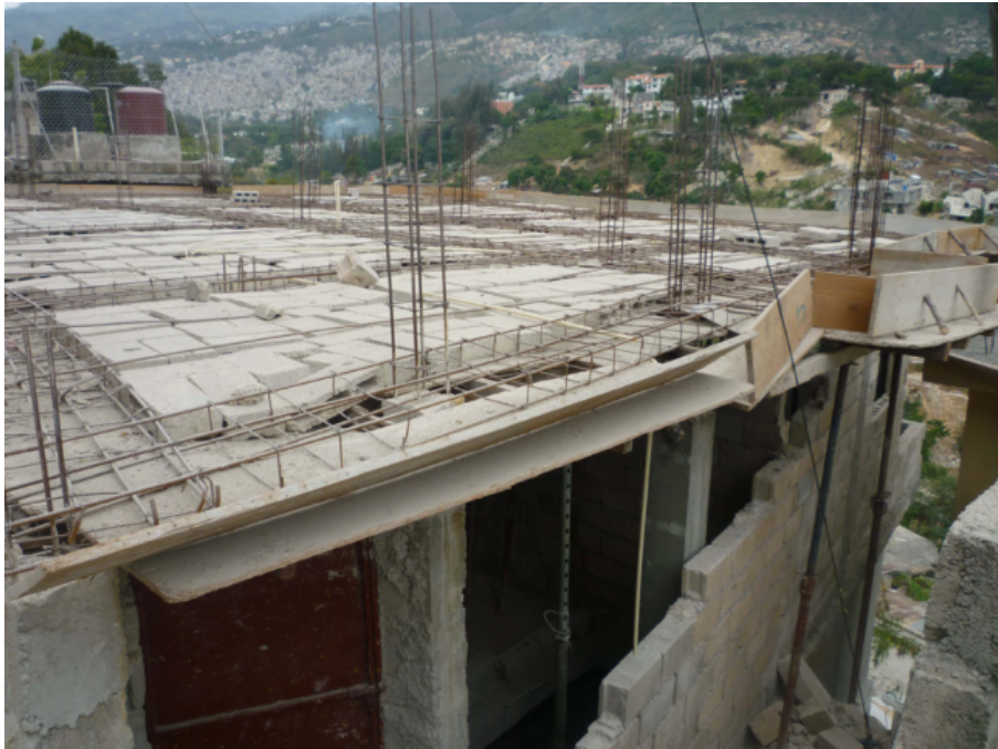
Figure 6.5: Building under construction in Haiti. Source DesRoches et al. 2011.
