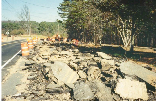
Figure 64. Full-depth pavement demolition.
