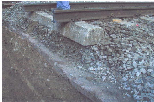
Figure 41. Asphalt layer beneath the ballast bed (Holzfeind and Hummitzsch, 2008).
