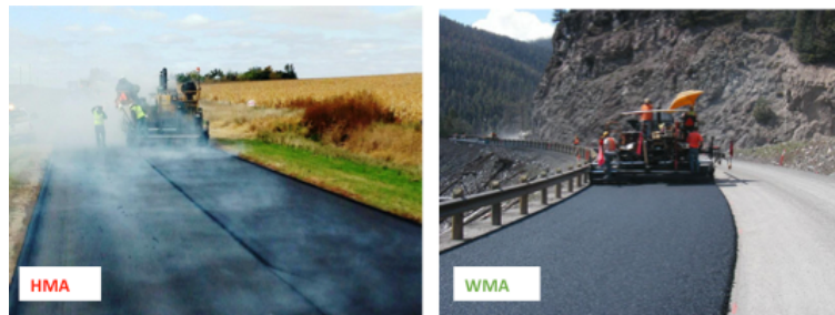
Figure 51. The fumes noted during the laying of HMA and WMA mixtures.
