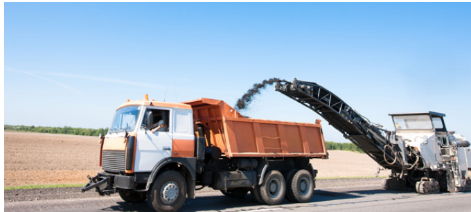
Figure 63. Milling machine removes asphalt pavement layers as part of pavement rehabilitation.
