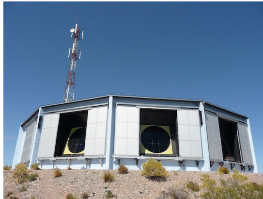
Figura 2.5: FD building at Los Leones during the day. Behind the building is a communication tower. This photo was taken during daytime when shutters were opened because of maintenance.
