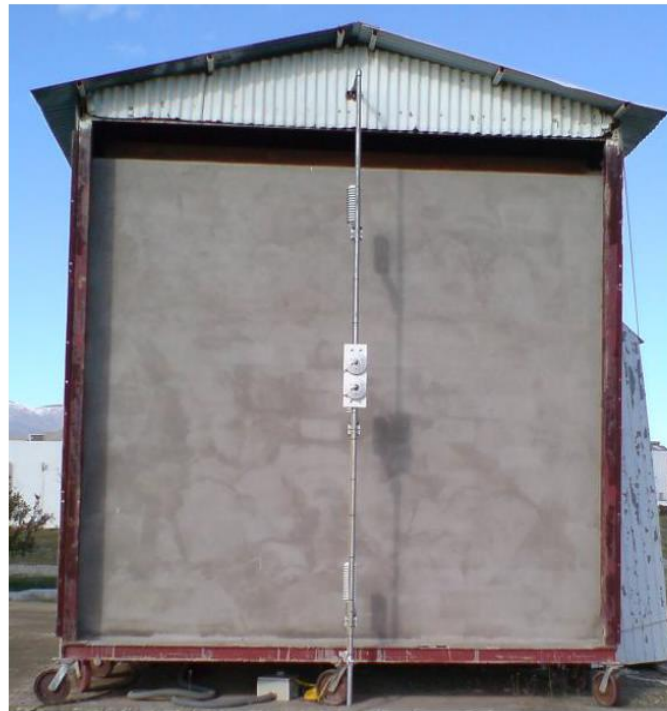
Figure 6.1. Exterior view of the test cell: wall tested with south orientation
