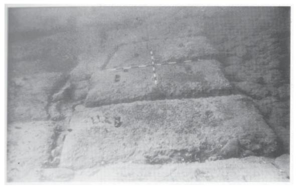
Image 25: Foundation blocks of the Jetty at Sidon (Frost 1975).
