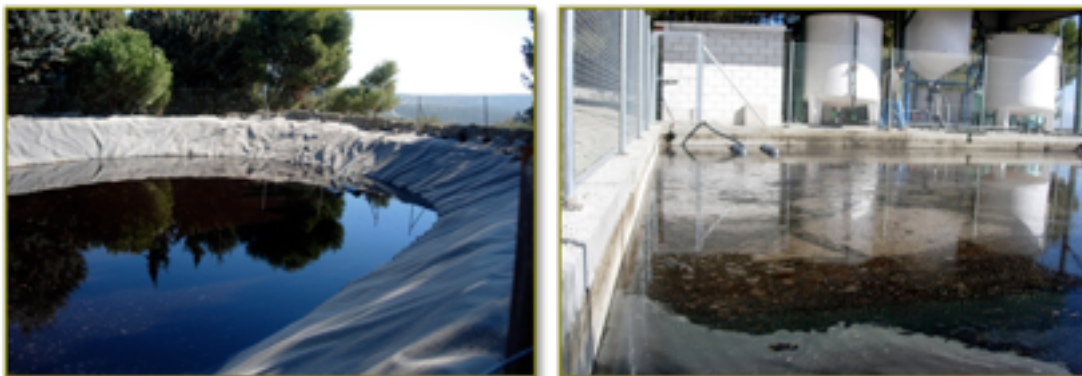
Figure 1.3. Artificial lagoons for storage and natural evaporation of OWW (left photograph) and OMW (right photograph).
