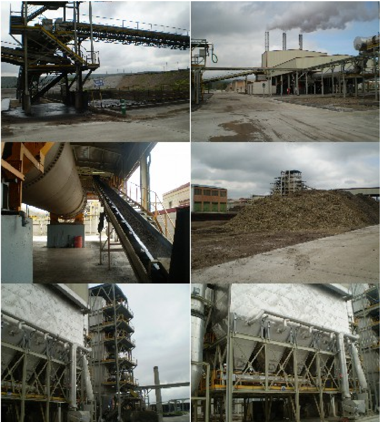
Figure 6.1. Pictures of the thermal power station in Linares (Southern Spain)
