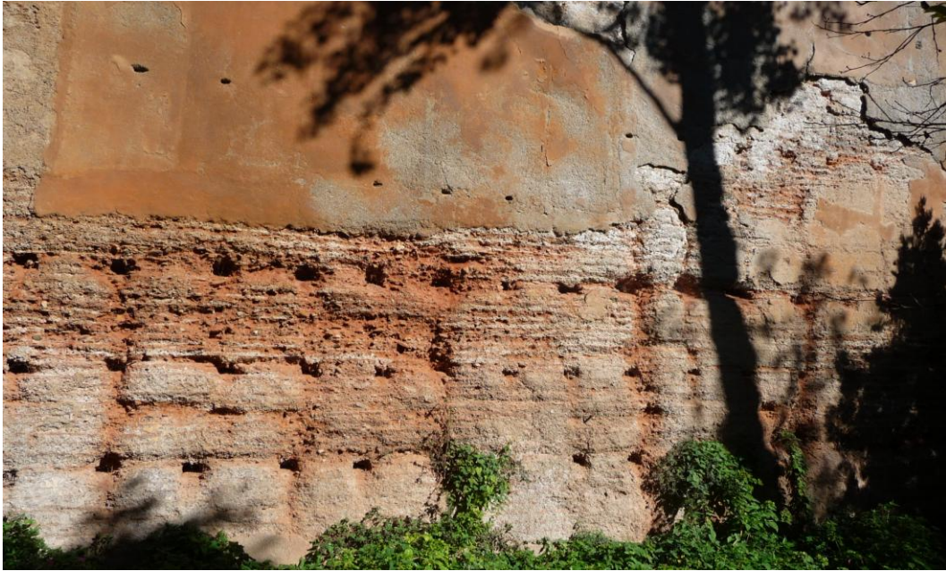
Figure 1-22. Tapial of the Alhambra. View from the "Cuesta de los Chinos", Granada, Spain.
