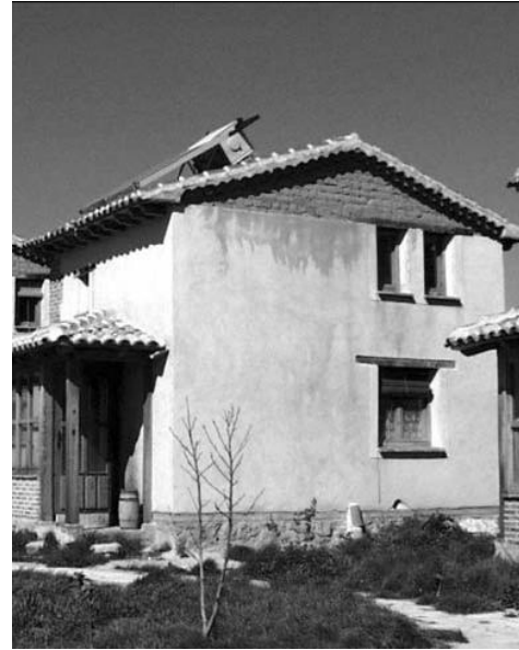
Figure 1-8. Earth walled house in ecovillage Amayuelas, Palencia, Spain (Jimenez Delgado and Cañas Guerrero 2006).
