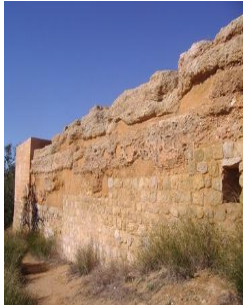
Figure 1-14. Rammed earth wall with rock foundation, Paderne Castle, Algarve, Portugal ( www.globedia.com ).
