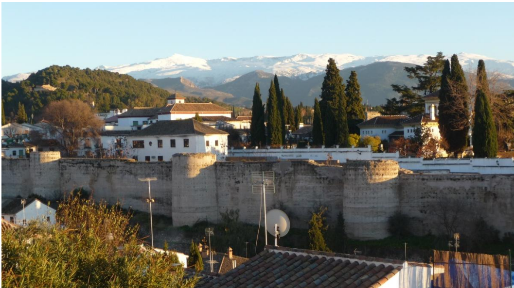
Figure 1-23. Historic city wall in the Albaizin, Granada, Spain. View from the "Mirador de San Cristobal".
