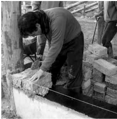
Figure 1-10. Construction of an adobe wall ( www.es.wikipedia.org ).
