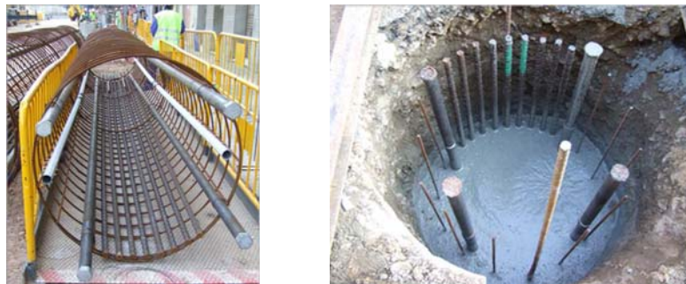
Fig. 1. Asymmetrical reinforcement for wall pile at construction site
