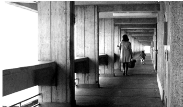
F63_ Bellefontaine, vista interior "coursive" grandes bloques, 1.972.CAPA
