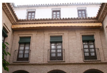
Ventanas Patio Interior
