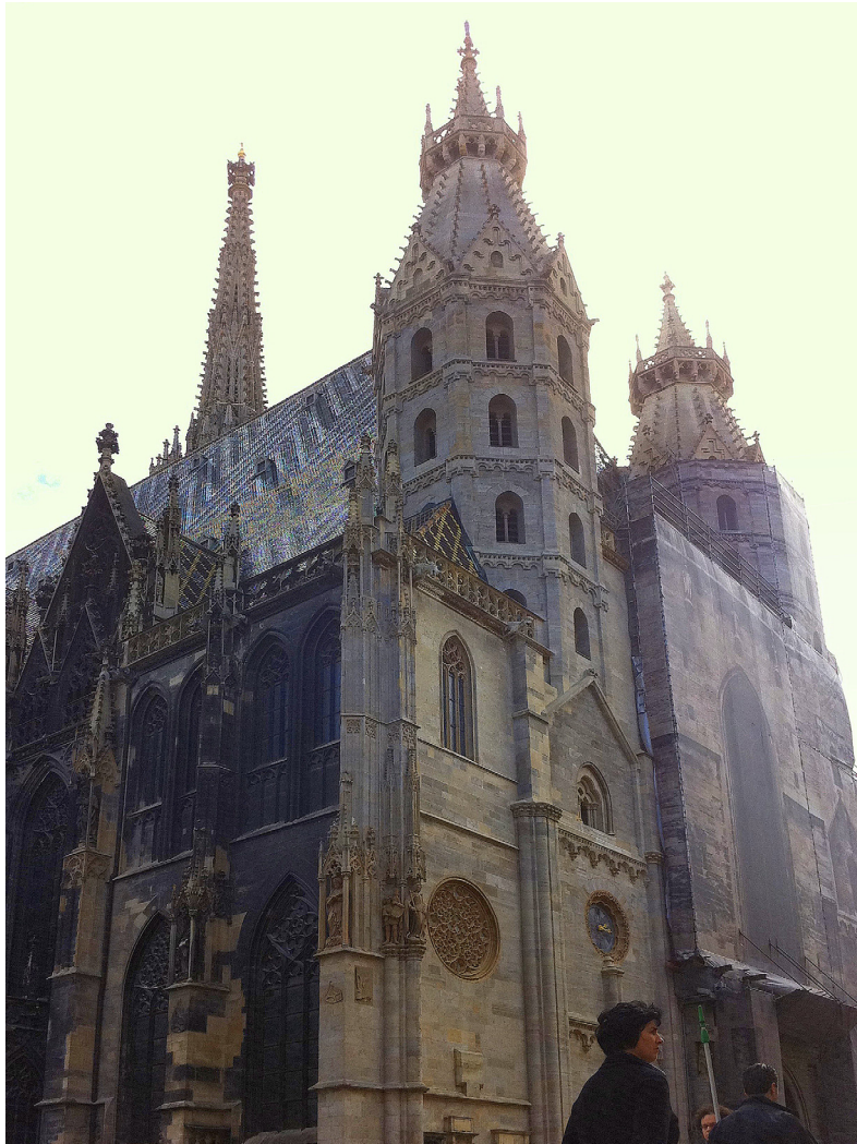
Figure 1. The restoration of the façade of St. Stephen's Cathedral (Vienna, Austria) is an outstanding example where optimal conservation procedures are essential to preserve the Cultural Heritage. Compare the restored (right) with the aged façade (left).
