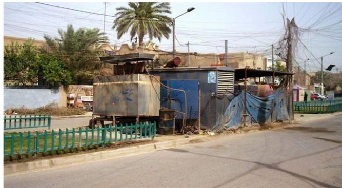
Figure 4.8: Installation site and cable routing of a NDG in an Iraqi residential area.
