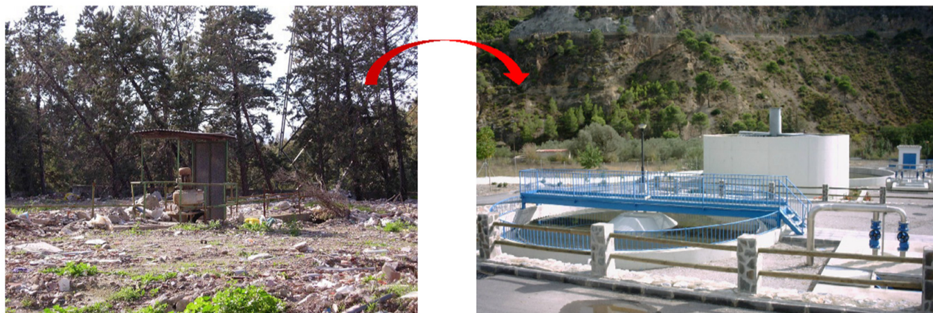
Figure 4. Water treatment plants in Órgiva. (Own elaboration). Note: Left: Old Órgiva WWTP using activated sludge technology, built in the 1990s and abandoned due to high energy costs. Right: New Órgiva WWTP using a bacterial bed system, built in 2004 and currently in operation.
