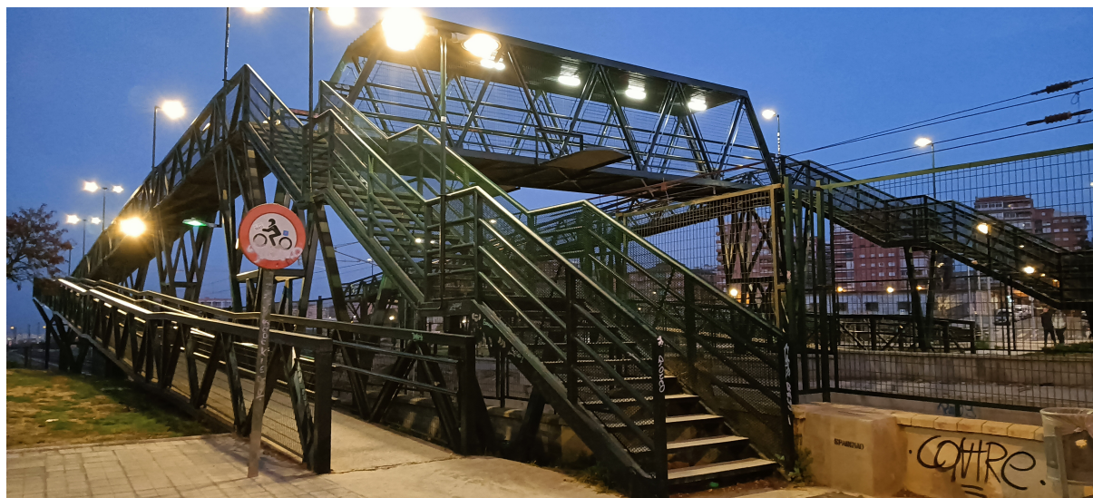
Figure 3.17: Case study 2: steel footbridge.
