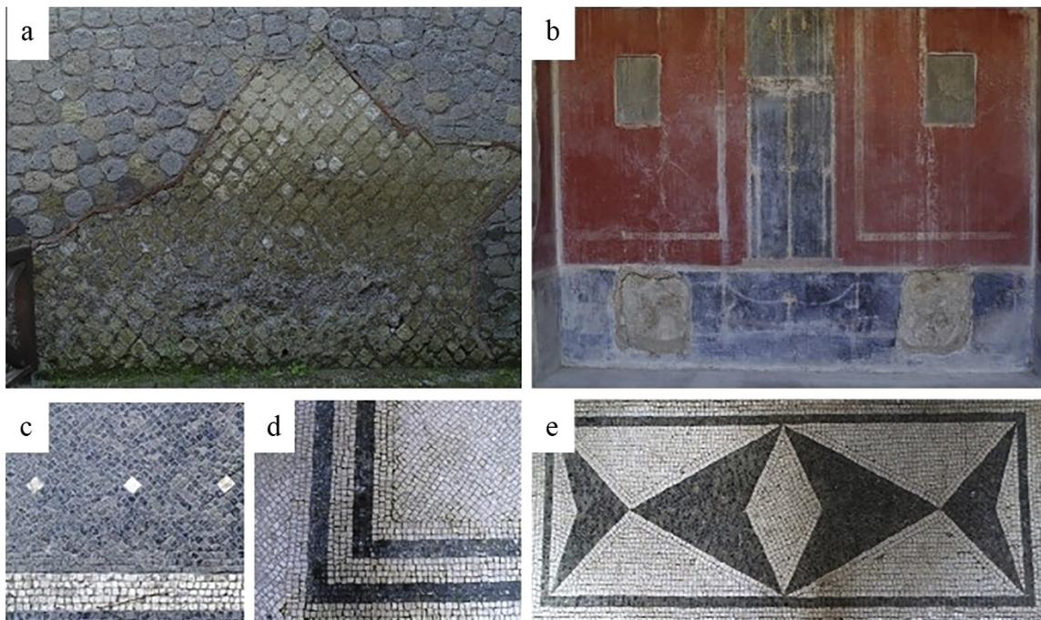
Fig. 3. Some architectural features of Villa San Marco: a) the original masonry in *opus reticulatum* separated by modern restoration; b) fresco mural painting realised in imitation polychrome orthostates; c), d) and e), geometrical shapes in mosaic floors.
