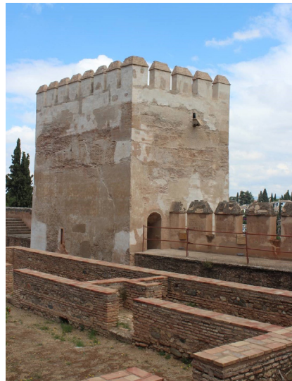
Figure 2: Restoration works on the Alhambra walls. Source: Alhambra Board of Trustees.
