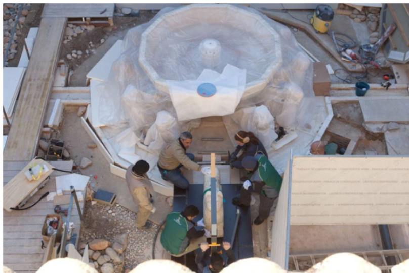
Figure 1: Restoration works of the Fountain in el Patio de los Leones. Source: Alhambra Board of Trustees
