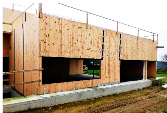
Figure 17. CLT construction. Health centre in Abegondo, La Coruña, Spain. January 2025.
