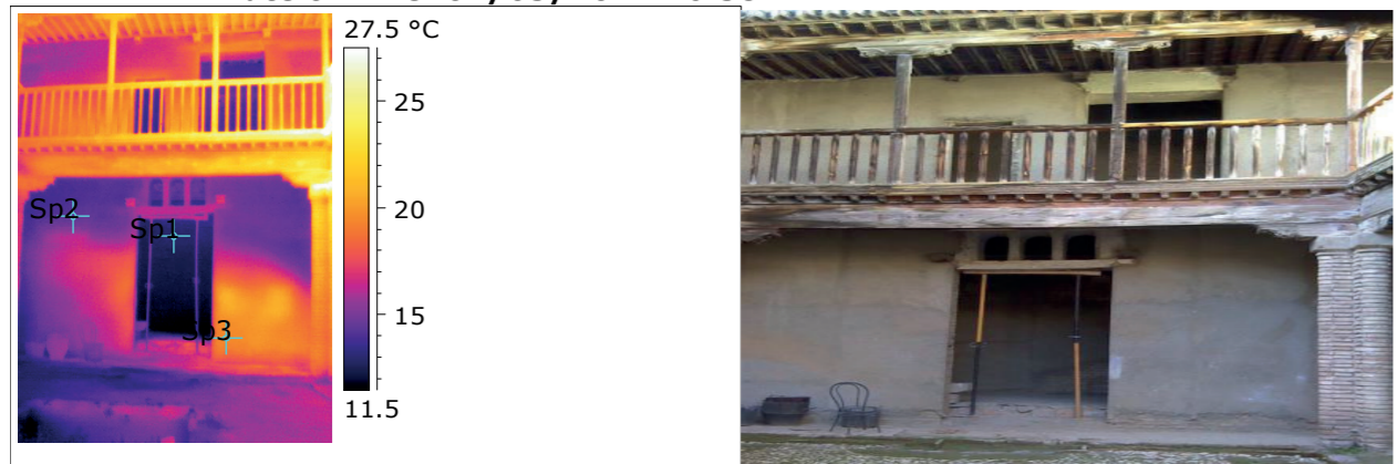
Picture 10. Captured at: Patio Date & Time: 07/03/2017 16:38:14
