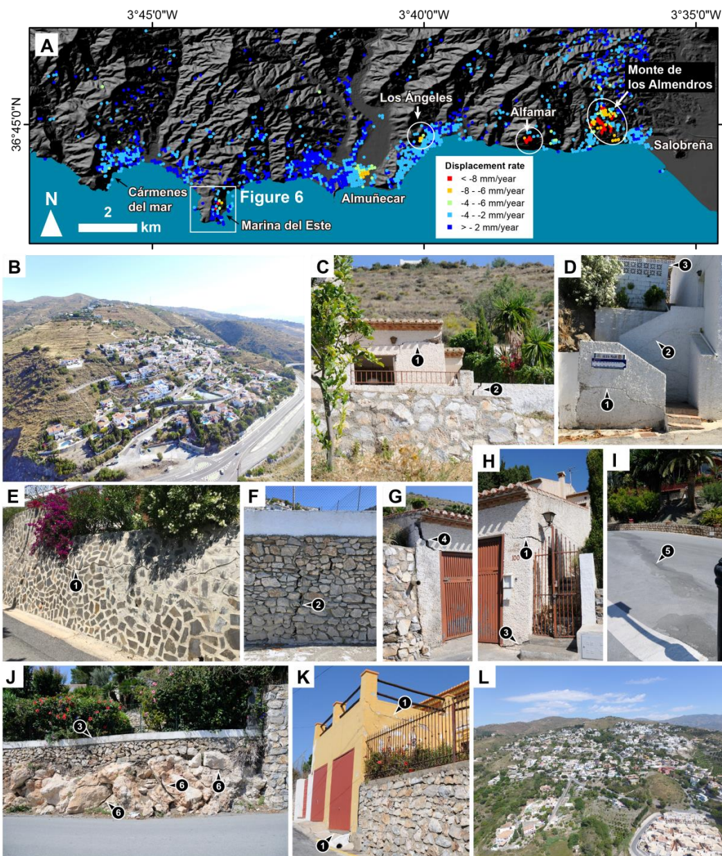
Figure 8. (A) GEP map data of the coast of the Granada province between the Los Cármenes del Mar resort and Salobreña. The urban states with ground instability problems are pointed out; (B) Aerial view of the Alfamar resort; (C–K) Types of damages observed in the Alfamar and Monte de los Almendros urban states. (1) Horizontal cracks on the top of buildings due to deflections of the slabs due to differential settlements; (2) Diagonal cracks and fissures due to foundation settlements; (3) Deformed walls; (4) Cracks due to deformation of the structure junctions; (5) Curved crack in the asphalt with a small step indicating differential settlement; (6) Open cracks in the bedrock; and, (L) Aerial view of the Monte de los Almendros resort.
