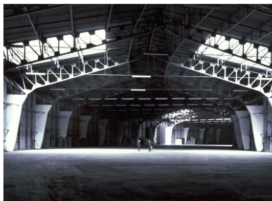
The cavernous Palace of Fine arts building before the Exploratorium moved in.
